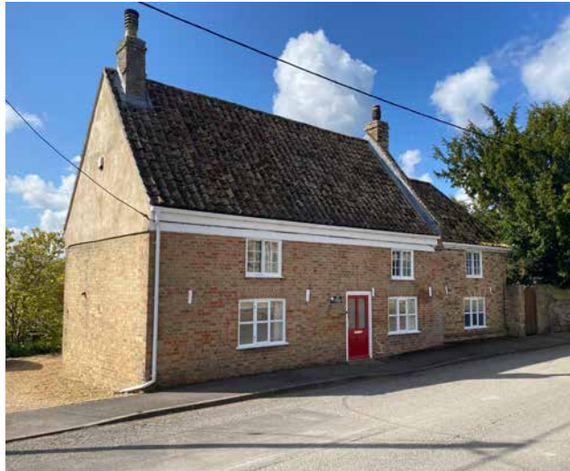
Figure 19: Listed property within the Conservation Area with no setback from the road.
