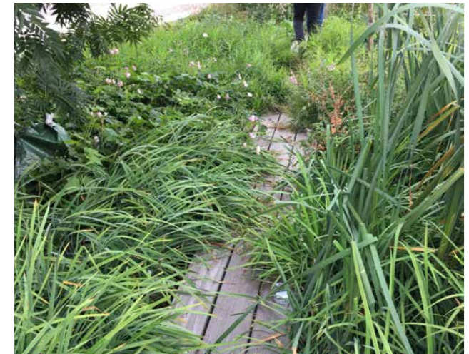
Figure 89: Examples of SuDS designed as a public amenity and fully integrated into the design of the public realm, Sweden. This is a 'rain garden' which is an intervention that can be used to enhance the capacity of the surface water piped drainage network by capturing and storing rainfall, allowing it to soak into the ground or release it slowly back into the piped network.
