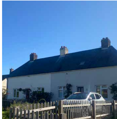
Figure 25: Typical semi-detached housing on Martins Lane.
