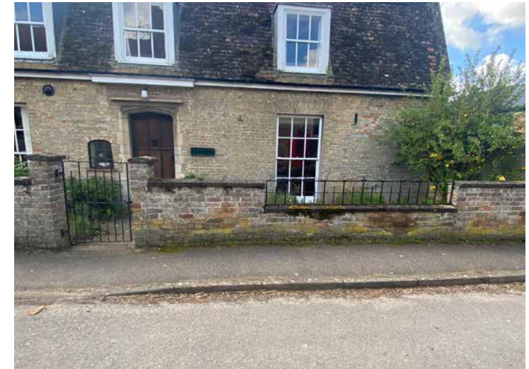
Figure 77: Low wall being used to define the boundary along the High Street which retains an active edge while creating an element of privacy.
