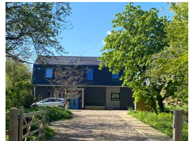
Figure 48: Passive house with on-plot car parking in Witcham.
