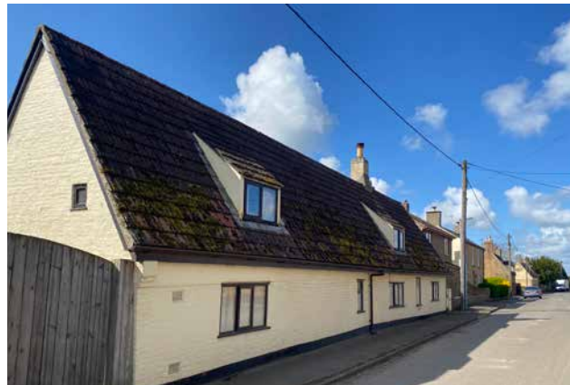
Figure 41: Linear style development with short or no setbacks in the Conservation Area.
