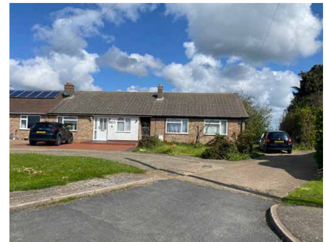
Figure 74: Bungalow in the Silver Street area.
