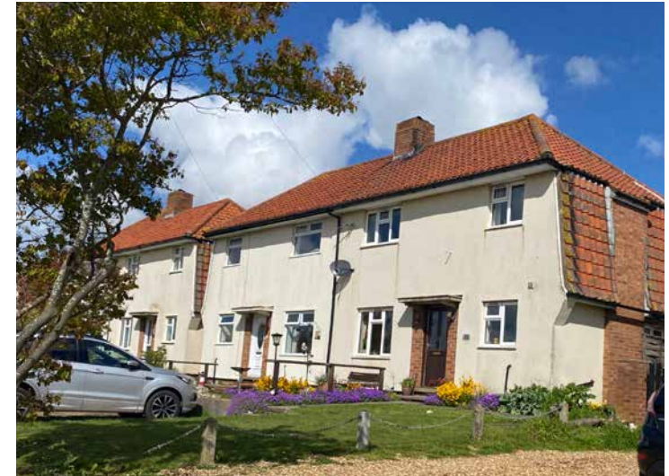
Figure 81: White render building with red hung tiles.
